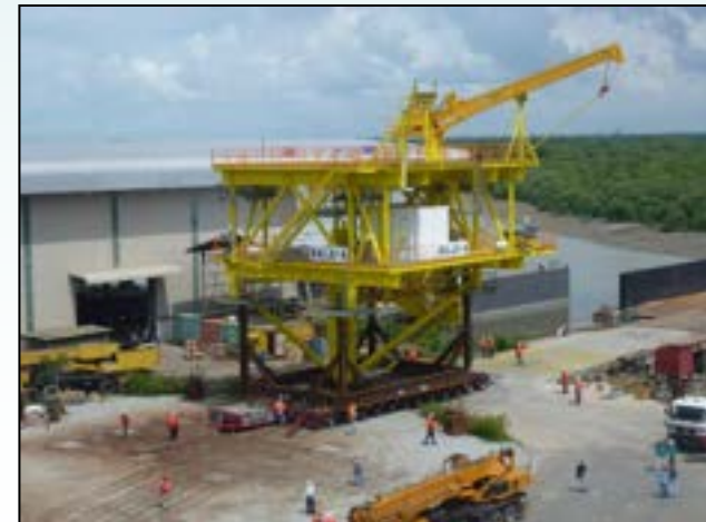
Balai platform load out
